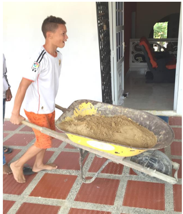
A Prosefam student helping to build the new school classrooms
